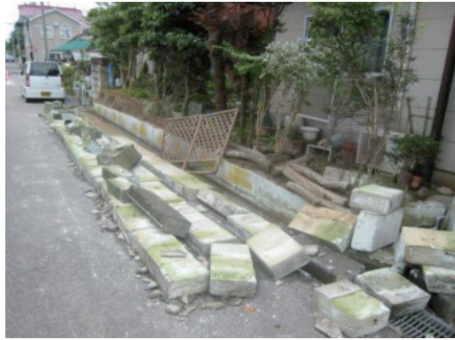
Collapsed stone wall
