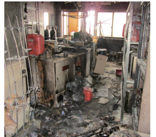
Traces of a fire of a chemical laboratory due to the shaking (in Tohoku Univ.)
